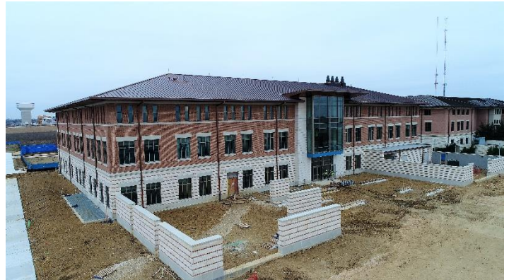
Rear Entry with Nursing in the background
