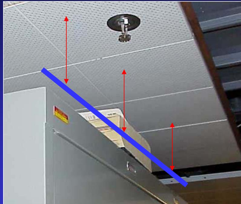
A simulated example of how storage can protrude into 18 inch plane below sprinkler heads.
