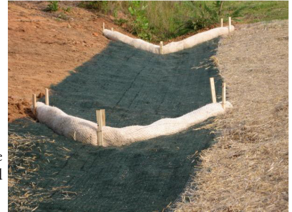
Jute erosion control fabric is coupled with straw wattles to minimize sedimentation. Photo by US Silt & Site Supply.
