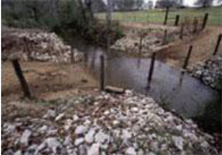
Livestock stream water crossing. Photo by NRCS.
