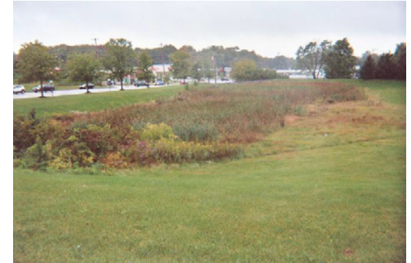
A naturalized & extended dry detention basin. Photo by F.X. Browne, Inc.
