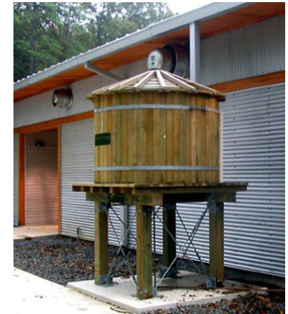
Seven hundred gallon rain cistern for the Camp Aldersgate Commons Building, Little Rock, AR. Photo by M.Littrell, Wilcox Group Architects.
