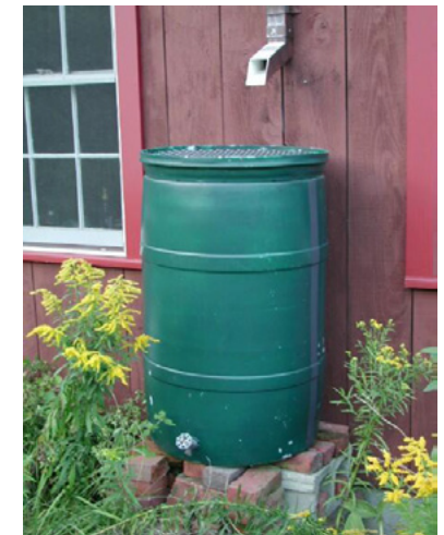
A rain barrel with sealed leaf/mosquito screen lid, spigot and connection to downspout. Photo by Lake County, IL Stormwater Mgmt. Commission.
