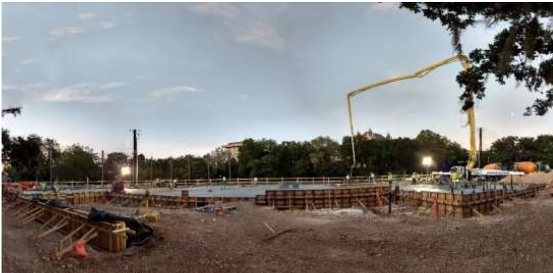
Foundation slab being poured
