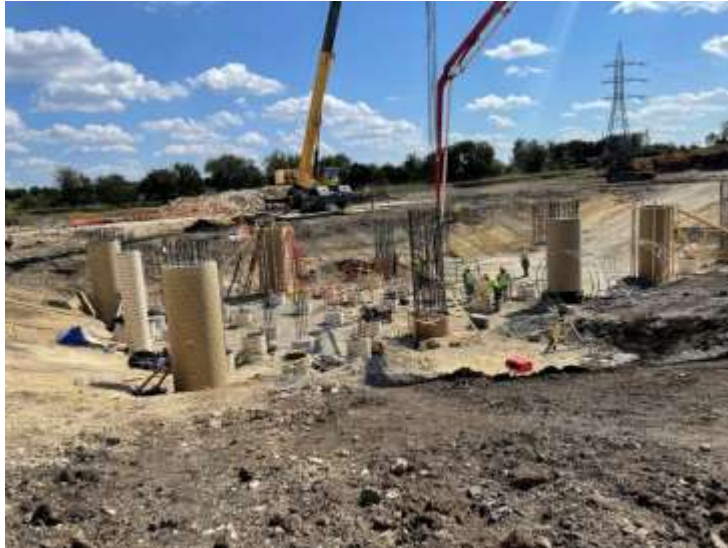
Basement foundation piers being poured
