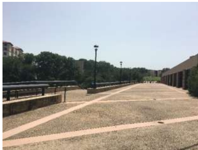
New Light Poles – Harris Dining Pedestrian Walk
