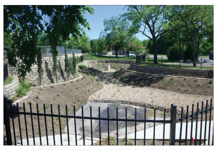
**Figure 2.** The completed Hutchison Biofiltration Pond (photo courtesy of Allyson Schlandt).
