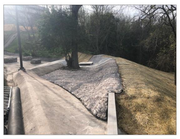
**Figure 3.** The completed Hogtrap Retrofit, showing the inlet before the piping goes below the surface. (Photo courtesy of Joey Kristoff)
