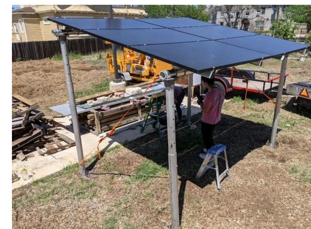
Figure 4: Final Assembly at Eco Centro in San Antonio, TX
